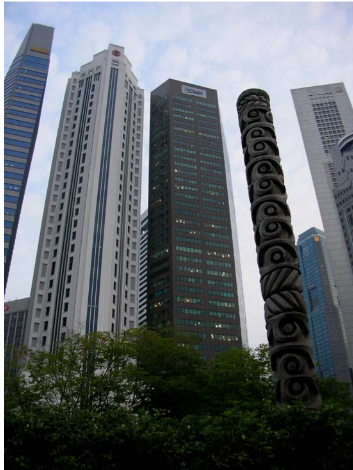
FIG. 8. Air-conditioned towers in Singapore – a country near the equator with high political transparency.
