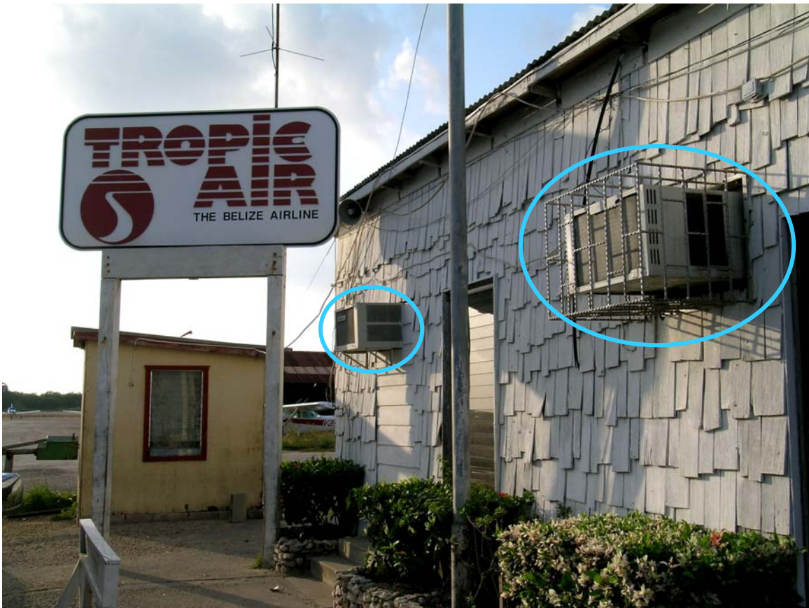
FIG. 8. Airline reservation office and terminal in Central America with requisite air conditioning.
