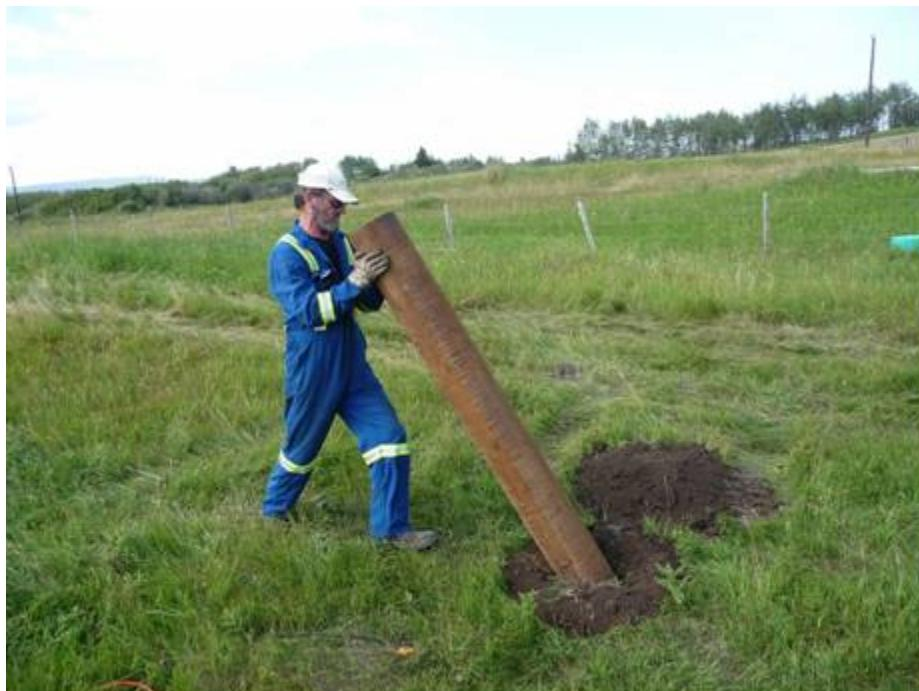
FIG. 9. Casing the shot holes.
