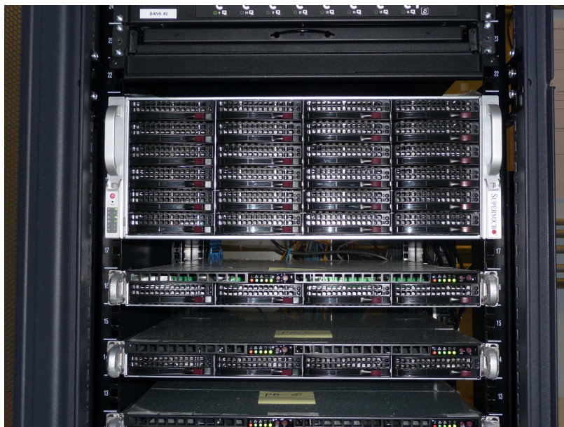
FIG. 4. Closeup of the master node and two side-by-side worker pairs
