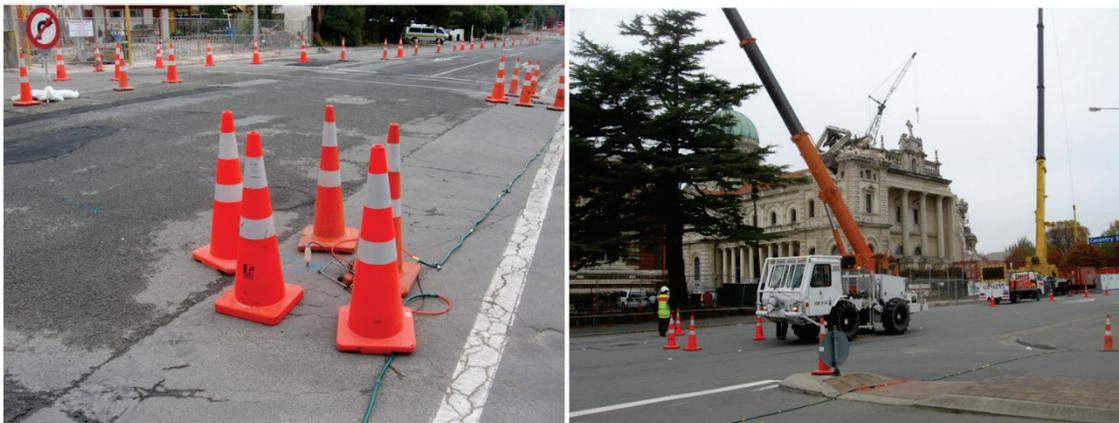
FIG. 9. Seismic acquisition along Barbadoes Street, Christchurch. Geophone plant (left) and source-point outside damaged Catholic Cathedral (right).
