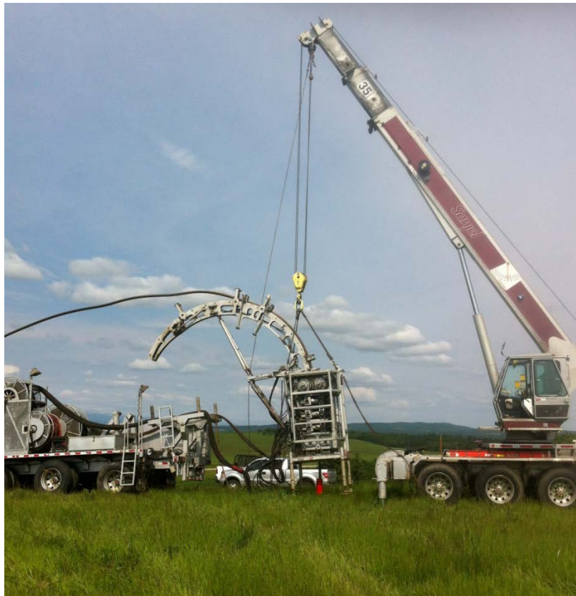
FIG 2. The coil tubing being inserted into Well 4.
