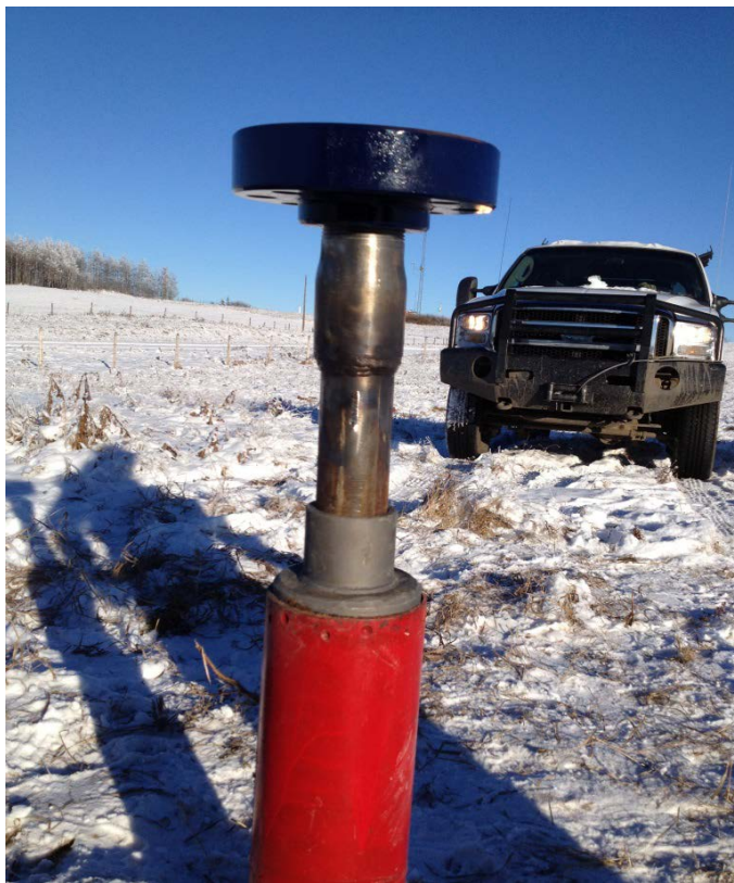
FIG 5. The finished coil tubing ready for the wellhead equipment to be installed.
