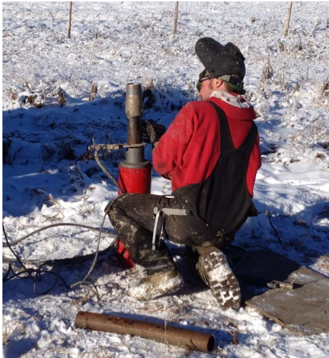
FIG 4. The bell nipple being welded onto the top of the coil tubing.
