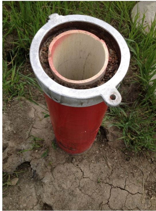
FIG 1. Well 4 before the installation of the coil tubing. The bentonite grout between the PVC casing and the steel conductor casing is visible
