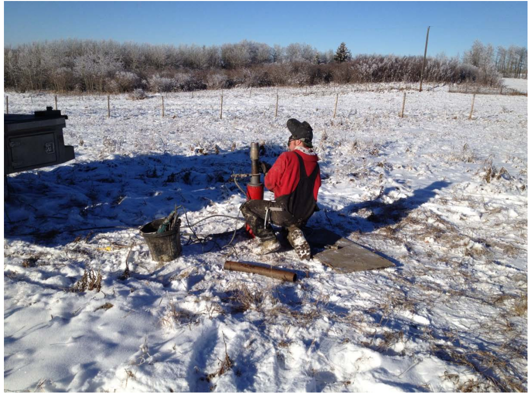
Preparing the top of the tubing for the well head installation 13 November 2014
