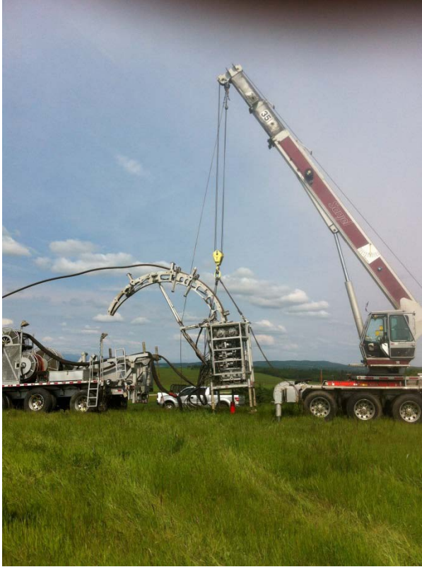
Installing the coiled tubing 30 June 2014
