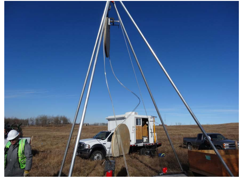
Installation of the cable in well 2
