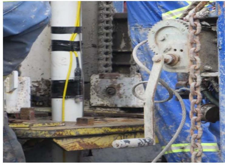
Installation of the geophones on the white PVC casing. The stainless steel tubing with the fibers inside is visible alongside the geophone housing. 11 of the yellow cables each have four 3C geophones connected. Cable 12 has a single 3C geophone giving 45 geophones overall. These are spaced at 3.06m from 11m to 146m. Following the insertion of the casing, the annulus of the well was cemented to surface.
