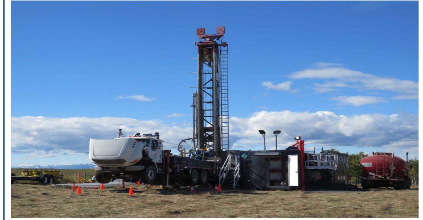
The drilling rig on site at Priddis. Two new wells were drilled in early October 2013. Well 1 is 146m deep and has 45 3C GS14 geophones installed on the outside of the casing as well as single- and multi-mode fiber for DAS recording. The reels of yellow down-hole geophone cables are visible on the trailer to the left.
