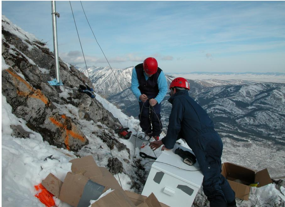
FIG. 4. Top photo: Installation of the mast on South Peak. Bottom photo: Installing mast and battery vault at the Third Peak station.
