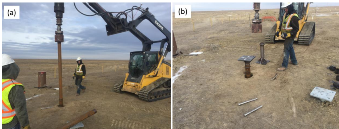
FIG. 4. (a) helical pile being installed at CaMI.FRS and (b) pile installed to a depth of 24.7 m with steel plate mounted on top of the pedestal (almost fully installed).
