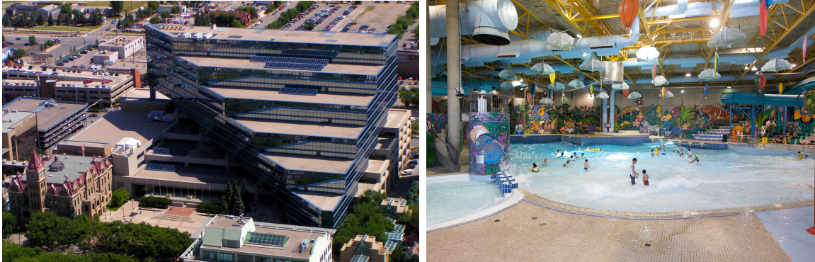
FIG. 20. Municipal Complex (left) and Village Square Leisure Centre (right).
